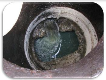
Bioaugmentation used for Grease & oil removal upstream in drains, channels & lift stations.
