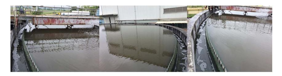
Unable to reduce BOD/COD sufficiently MicroBlock used upstream in lift station Bacteria and Micronutrients used in MLSS
