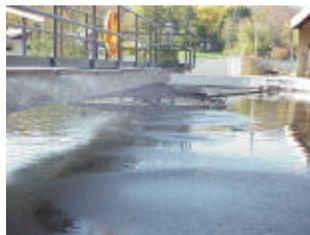
If need be, add a sprayer to your clarifier if your clarifier is old, and you do not have the capability to completely handle the solids. The weight of the water alone will knock down any solids and help with gassing, ashing and high effluent TSS.
