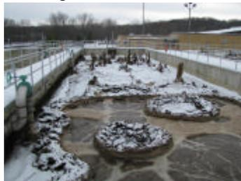
Frozen ice towers in a digester are shown below; this was an interesting phenomena. The bubbling action of the diffusers caused small formations to slowly build up and freeze.
