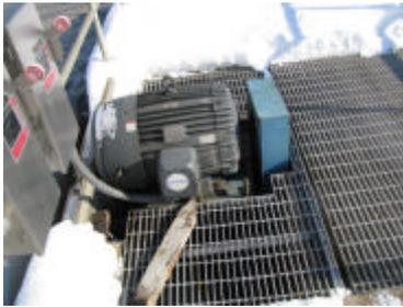
Build-up around pump and aerators can make mechanical equipment harder to run or easier to break down.
