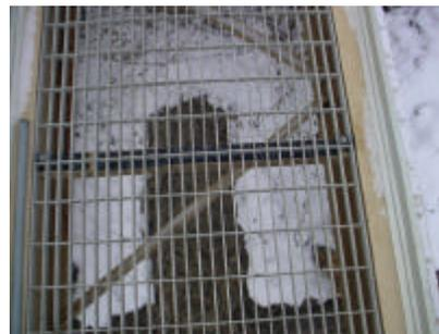
Channels can freeze up and block the flow
