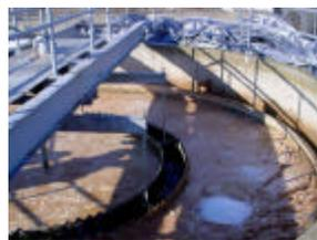
Whether it is in the aeration basin, channels or in the clarifier, foam and filaments due to grease rises to the surface, does not mix well, sits there longer and eventually freezes on the surface.
