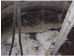
Grease trap sizing criteria are typically based upon old regulations written when animal fat was the main form of cooking oil used in kitchens. Nowadays there are modern oils or liquid oils that remain liquid at room temperature, and may be more
