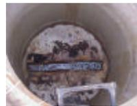
Most blockages and sanitary sewer overflows in wastewater collection systems are caused by grease. As the temperature cools down in the winter, wastewater from toilets, kitchen sinks, and other sources flow more slowly to the wastewater treatment plant. As a result, grease and other household products tend to harden and collect in cold sewer pipes, causing blockages and occasional
