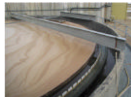
Clarifier with foam carryover from Aeration basin,
