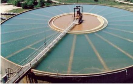
The reaction of lime with phosphate is pH dependent. The solubility of hydroxyapatite is low. At a pH of 9, a large fraction of the phosphorus can be removed. In lime treatment of wastewater, the operating pH is often determined by the pH required to obtain good suspended solids removal, and as long as pH exceeds 9.0, good phosphorus removal will generally follow.
