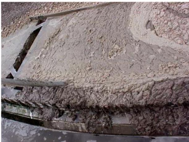
Holding solids too long generally causes not only septic conditions, which can generate odors, but also generates low DO conditions which can generate specific compounds with sulfides and/or organic acids. Limited nutrients are available also to the bacteria in the clarifier. All of these conditions promote the growth of filamentous bacteria. Holding times of influent should always be kept to a minimum. Generation of septic conditions can also contribute to
