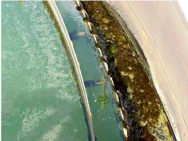
This clarifier and the draw down mechanisms will have to be checked and cleaned out during scheduled maintenance. The appearance of the surface of the sludge thickener tank showed too much water, which also might indicate "rat-holing" occurring in the clarifier.
