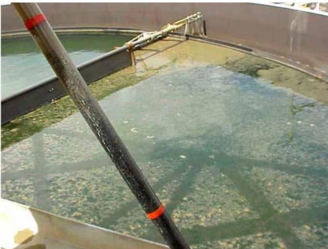
During a training class of 12 operators, we had them all pull a sludge judge to see if every operator pulled it at the same spot in the clarifier and pulled it at the same time according to the position of the rakes.
