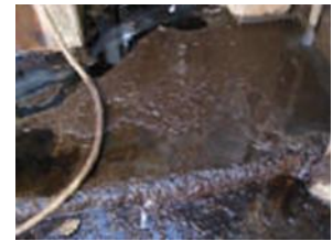
Blocked sewer with oil build-up Oil leaking off machines
