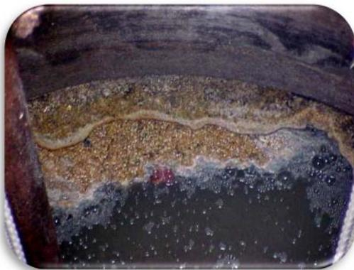
What are signs that the product is working- Foaming in the lift station- white foam at first shows the bugs are in a high growth phase, as the foam turns to a light brown, they are getting a little older.
