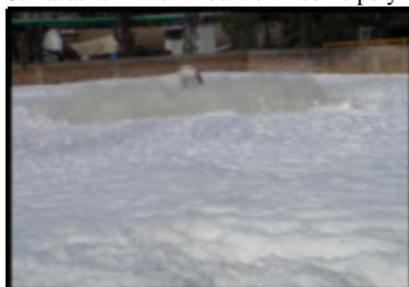
Excessive foam, especially in an aeration basin, can cause a variety of problems. A foam blanket on the aeration basin can interfere with oxygen uptake of the microorganisms and hinder BOD reduction. Foam can also cause the
