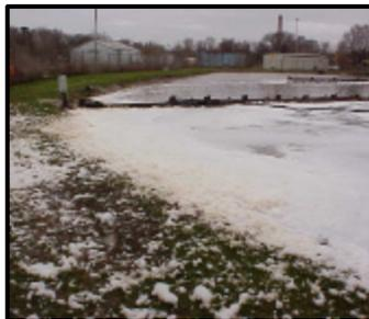
Antifoams control or eliminate foam in secondary treatment or final effluent areas of a waste treatment plant. Reducing foam by using antifoams in the past has been desirable for safety, health, and aesthetic reasons. Controlling the source of the foaming is usually a cheaper and better solution long term.
