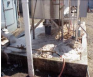
Very young sludge at a winery, spilling out of equipment - Young sludge at meat packing plant - surfactants in DAF upstream causing some of the foaming also
