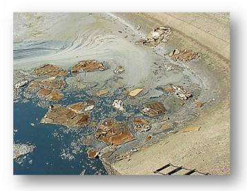
filamentous sulfur bacteria, toxicity, etc. Aeration oxidizes H2S to odorless sulfur species, generating either free sulfur or sulfate. pH modification establishes basic pH conditions (7.5-8.0) so that the majority of the sulfide occurs in the odorless hydrosulfide ion form (HS-).
