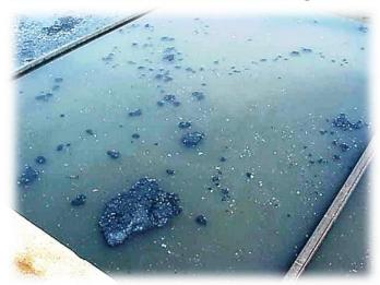
On the left is a secondary clarifier with solids build up on the support structures. Ashing and Gassing is present. Make sure to clean side walls, struts, center wells as well as make sure the solids on the
