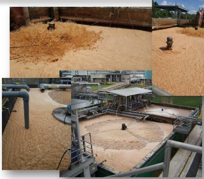
Pharmaceutical plant with high foaming and zooglea in anoxic and aeration basin After addition of Bioaugmentation MicroSolv 200 and MicroClear M100 micronutrients and adjustments to N and P values.
