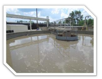
After addition of Bioaugmentation MicroSolv 200 and MicroClear M100 micronutrients and adjustments to N and P values.
