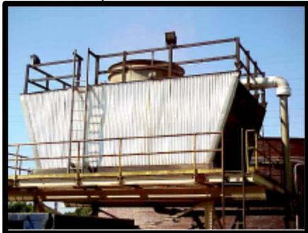
that are kept open, meters, Water softener, make up water, RO filtrate, condensates, holding tanks, wet wells, pits, storm water. Boiler Blowdown: The use of boiler blowdown as cooling tower makeup is another reuse scheme that has been employed at a number of locations.
