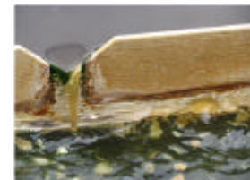
and final effluent red from overdose of Ferric
