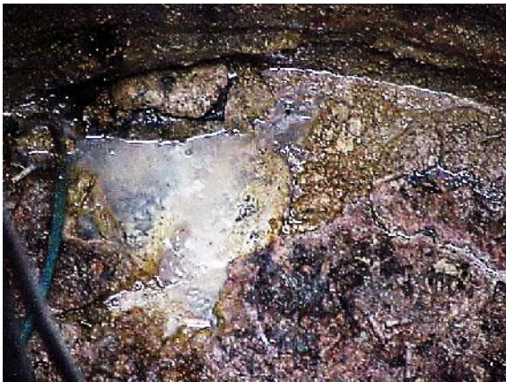
Lift station filled with grease
