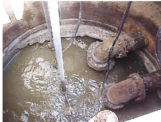
Lift station after short use of bioaugmentation
