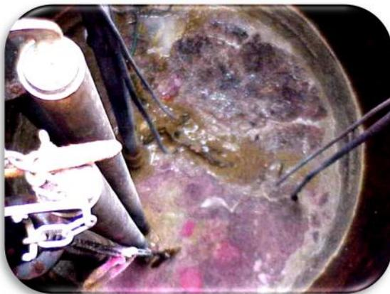
Application of product is improper here, pink product all over the top of the grease and not really in contact with the water
