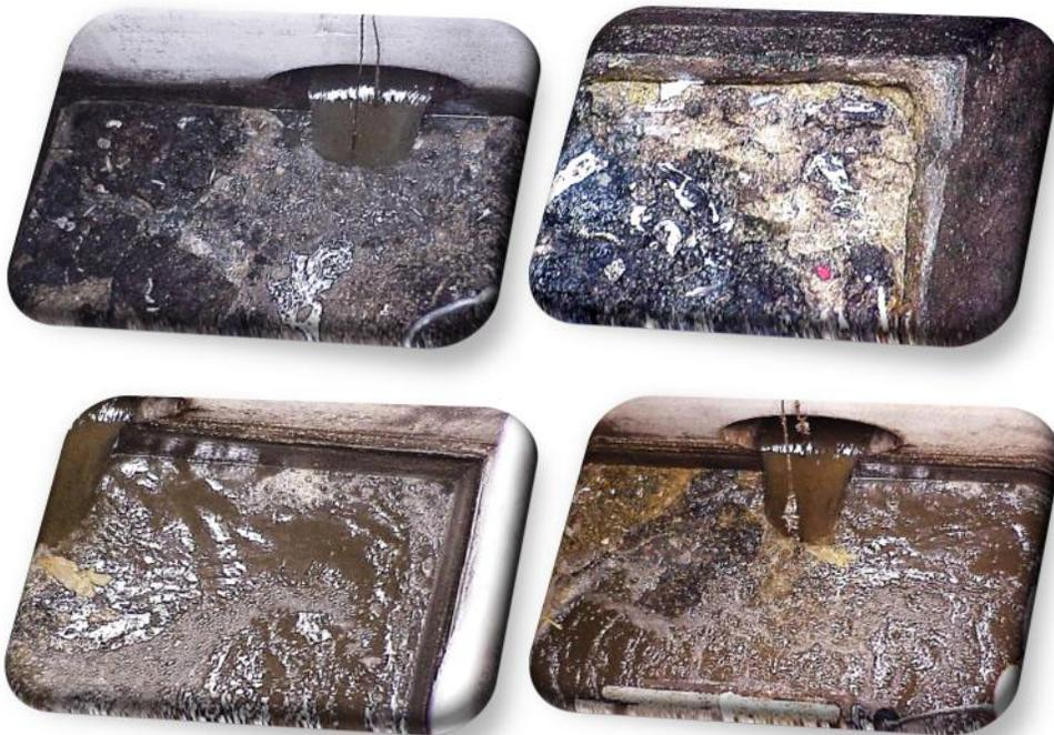
This lift station in top 2 images, before bacterial product (bioaugmentation) was introduced. There were thick solids built up in the corner & grease crust ledges.
