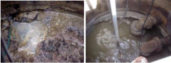
Lift station filled with grease
