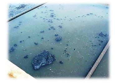
On the left is a secondary clarifier with solids build up on the support structures. Ashing and Gassing is present. Make sure to clean side walls, struts, center wells as well as make sure the solids on the
