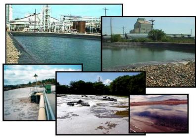
Lagoons come in all sizes and shapes. A lagoon can be a stabilization pond, an aerobic lagoon, High-rate aerobic pond, Low-rate aerobic pond, Maturation or tertiary pond, Facultative pond, Facultative pond with mechanical surface aeration or an anaerobic pond.
